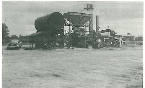
Here is the new asphalt plant at Monticello which was rebuilt and remodeled by J. L. Goins and his mechanics.
